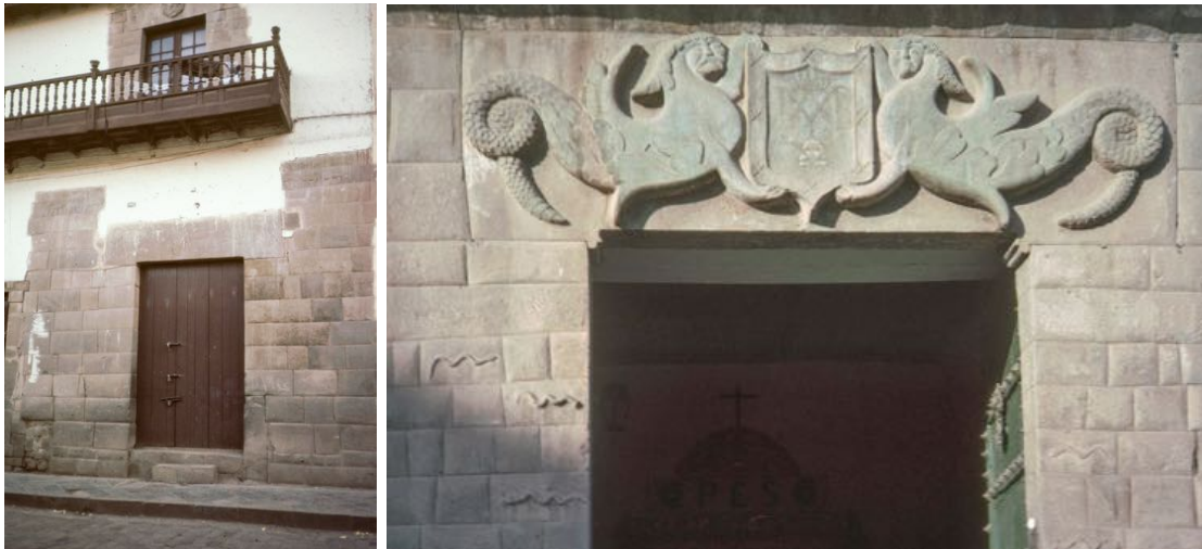
Figure 1066. Colonial houses built upon indestructible Inca foundations.
