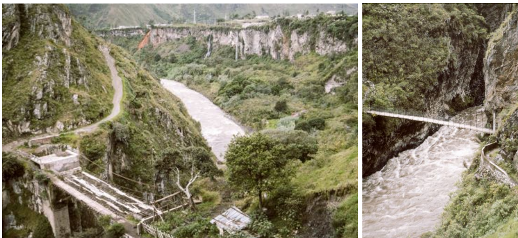
Figure 995. Bridges across the Río Pastaza.
