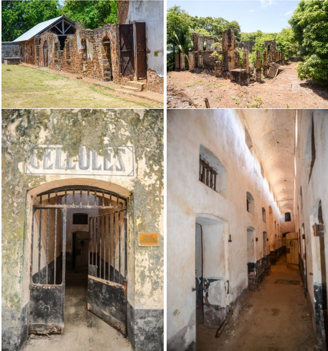
Figure 1049. Row of cells and a building recovered by nature, cellules (cells) with stands for iron bedsteads.
