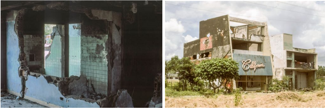
Figure 705. Former bathroom and former cinema.
