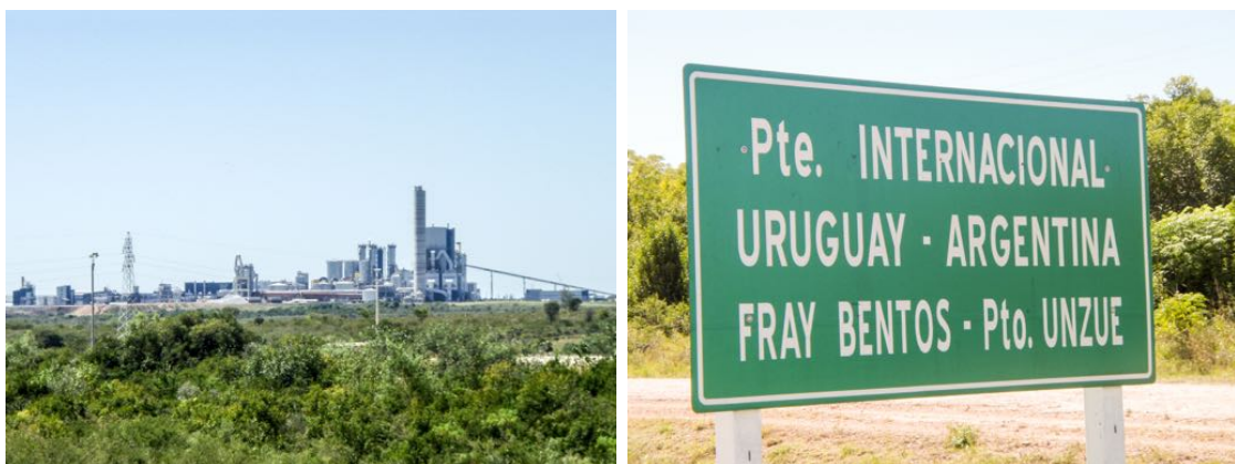
Figure 1434. Finnish pulp factory from a distance, and the International bridge .
