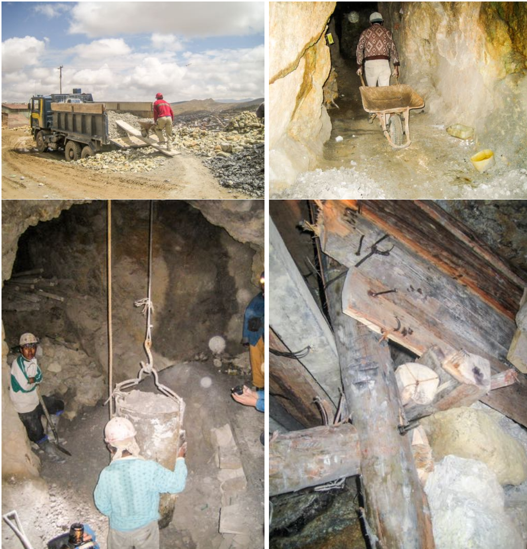
Figure 1161. Emptying a wheel barrow and pushing it back inside the mine. Workers in the mine and a rusty clapboard construction holding up the roof.
