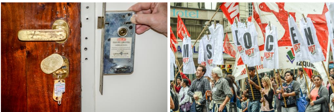
Figure 1409. Our broken door lock. Demonstration in Buenos Aires.
