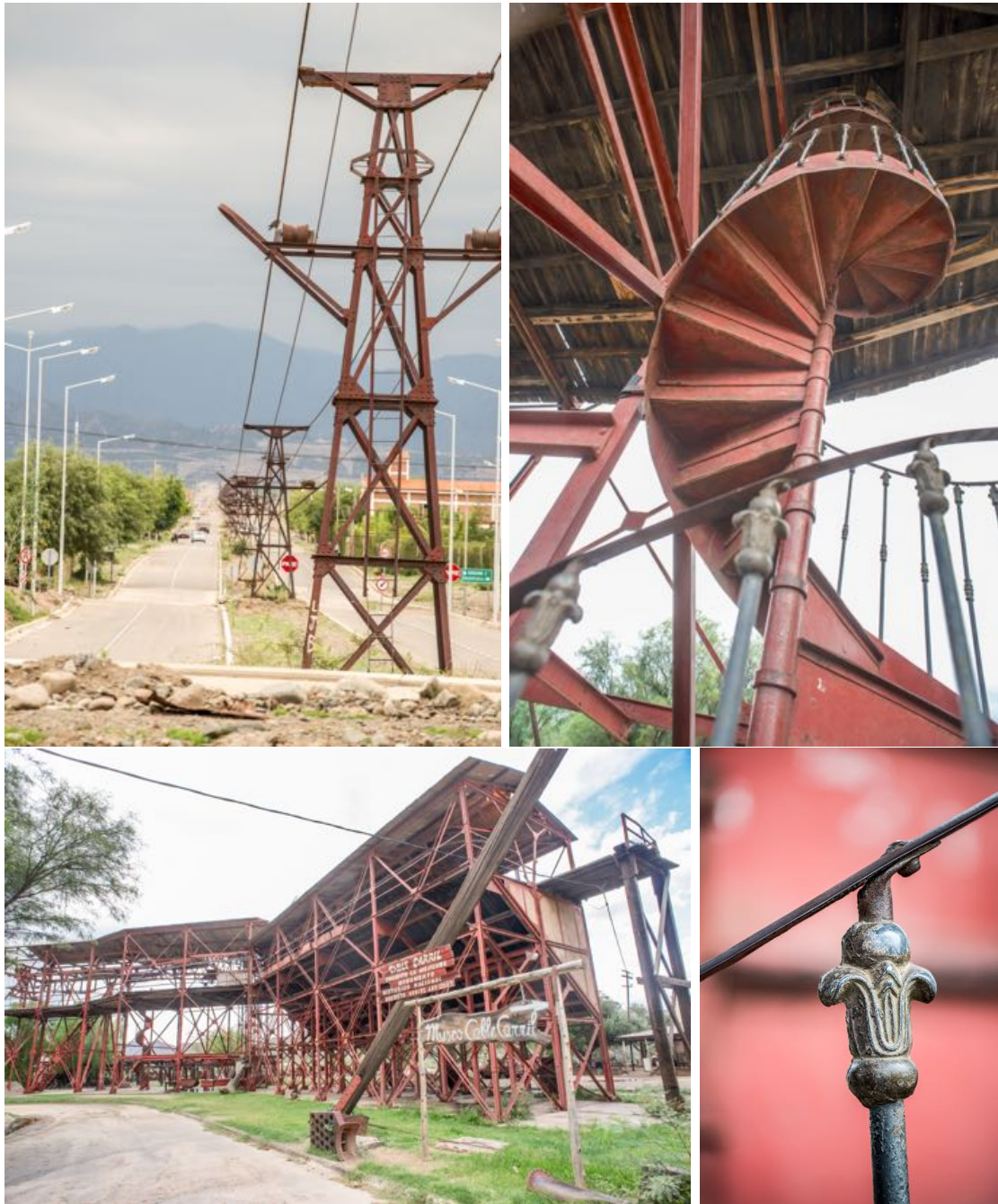
Figure 1359. Chilcito cable car.
