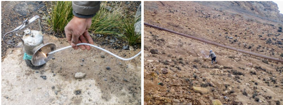
Figure 1165. Lighting the fuse and exploding the dynamite at a safe distance.
