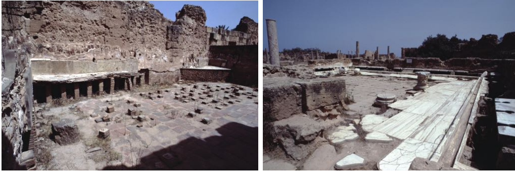
Figure 109. Leptis Magna: Roman baths. Hot air circulated between the brick columns under the raised floor.
